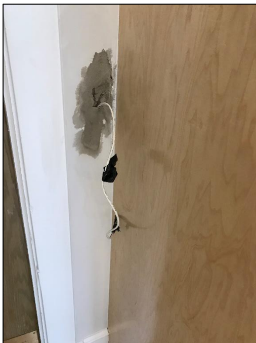
Room 10 – Exposed wires near door.
