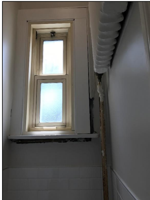
Room 8 – Exposed radiator piping and missing trim.
