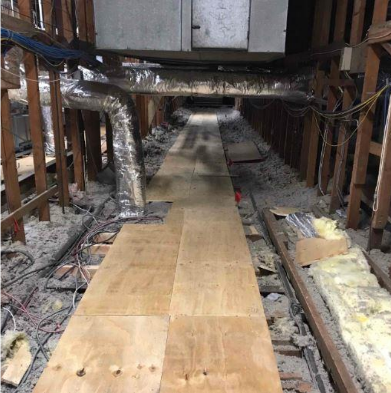
Construction of Proposed Attic Platforms at Edgewood & Fox Meadow
