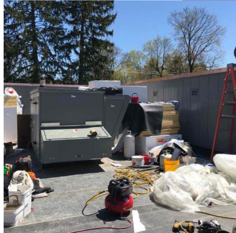
Installation of New Addition HVAC Roof Top Units
