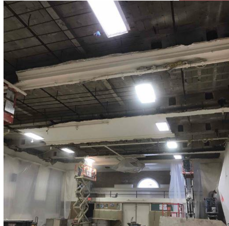
Demolition of Existing Gymnasium Ceiling to Facilitate Proposed Skylight Openings.
