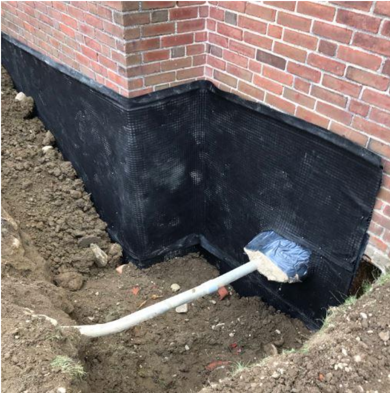
Installation of Foundation Wall Waterproofing at Quaker Ridge ES
