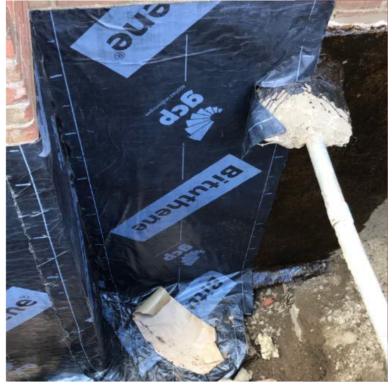
Installation of Foundation Wall Waterproofing at Quaker Ridge ES
