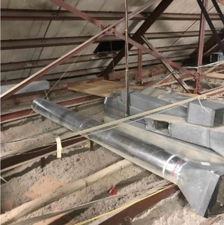
Demolition of Existing Attic Duct Work at Edgewood & Fox Meadow
