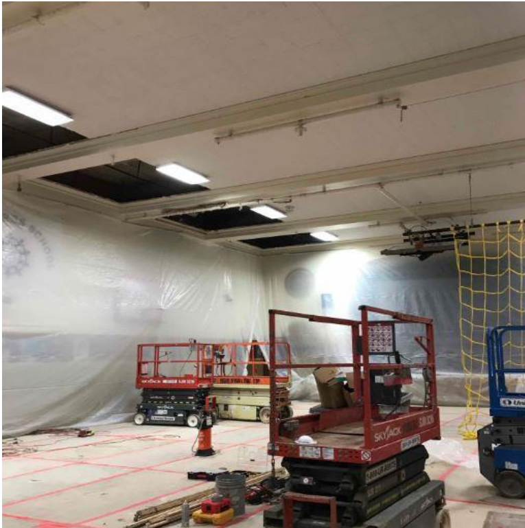
Demolition of Existing Gymnasium Ceiling to Facilitate Proposed Skylight Openings.
