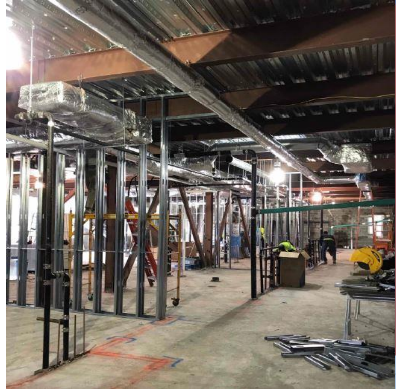
Light Gauge Metal Framing at 2 nd Floor of New Addition
