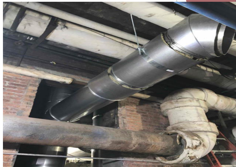
Construction of New Boiler Breaching
