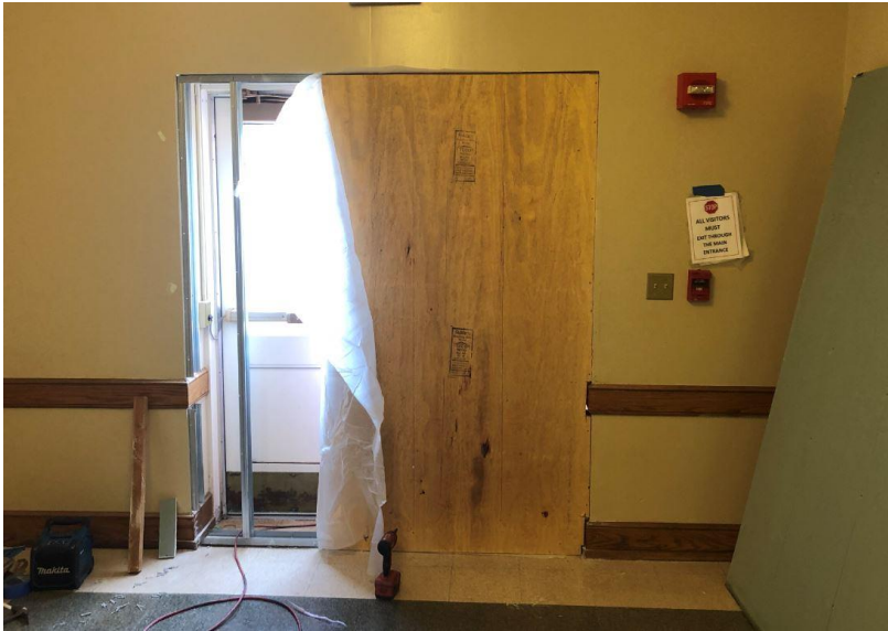
Construction of Temporary Partition
