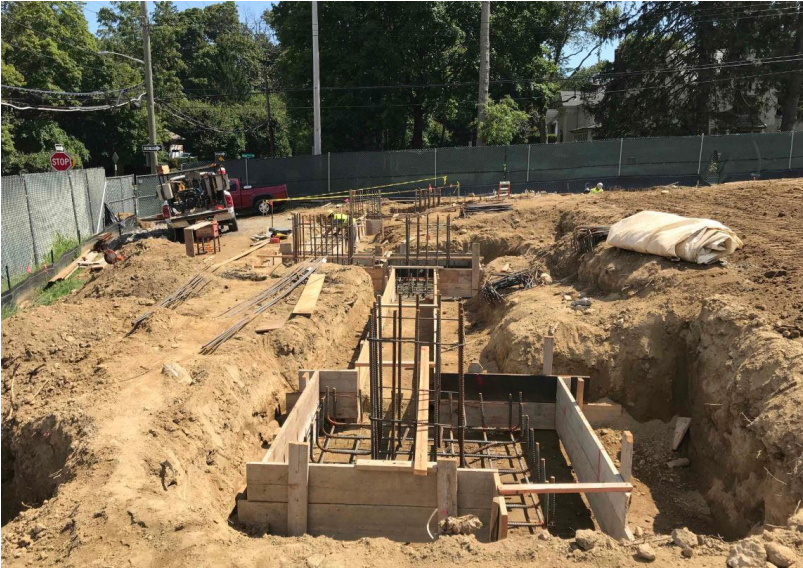
Construction of Proposed Addition Footing Rebar and Formwork
