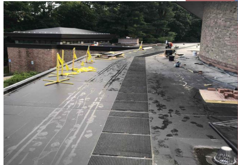
New Roofing System and Walk Off Mats
