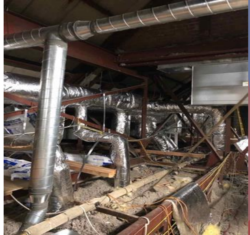
Installation of new duct work within existing attic (E.W.)
