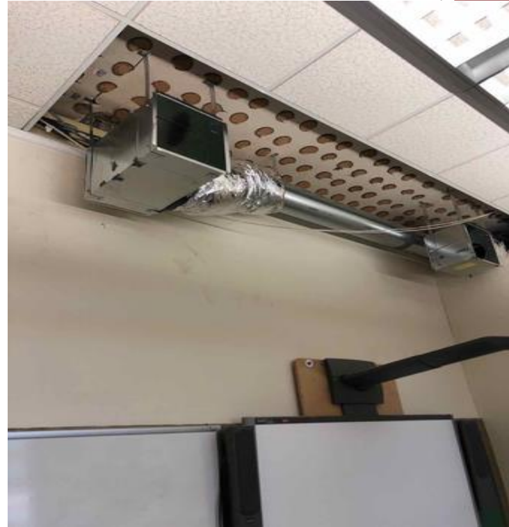
Installation new duct in classroom (F.M.)
