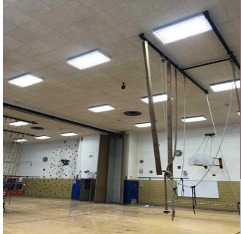
Installation of new ceiling grid and tiles, and lights within Middle School gymnasium.
