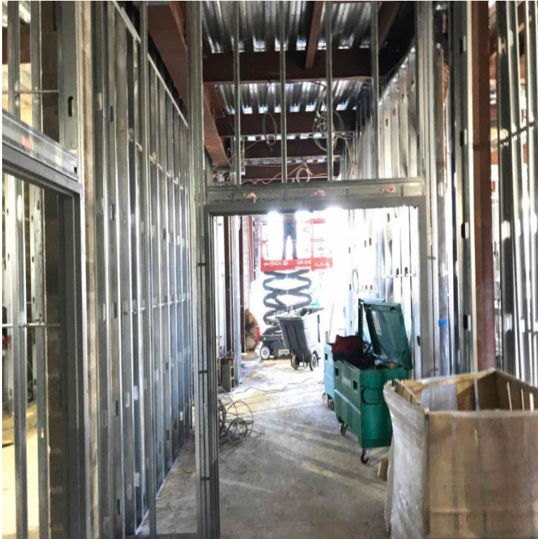
Construction light gauge metal framing interior partitions at Corridor 144 (adjacent to MPR Room)
