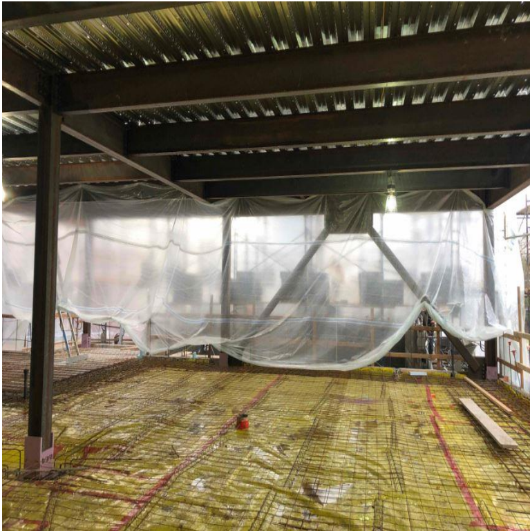
First floor slab on grade preparation
