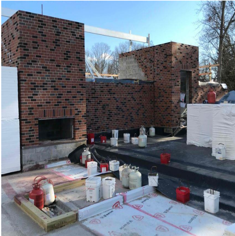
Installation of EPDM roofing system above Learning Commons and MPR areas.
