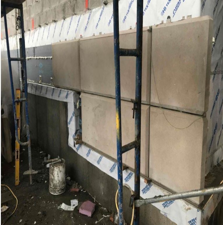
Construction of exterior cast stone panels
