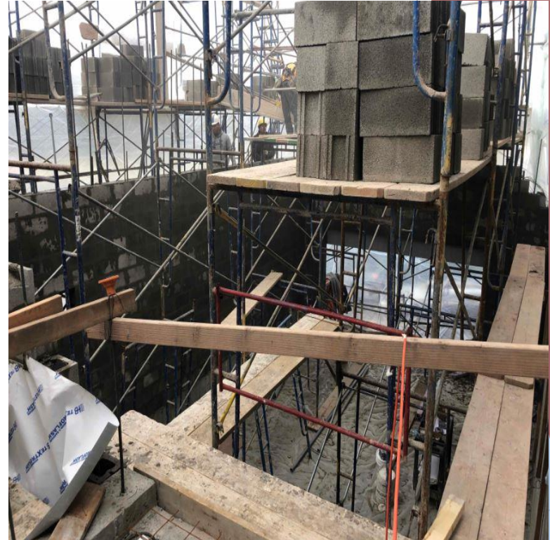
Construction of stairwell 163 CMU partitions
