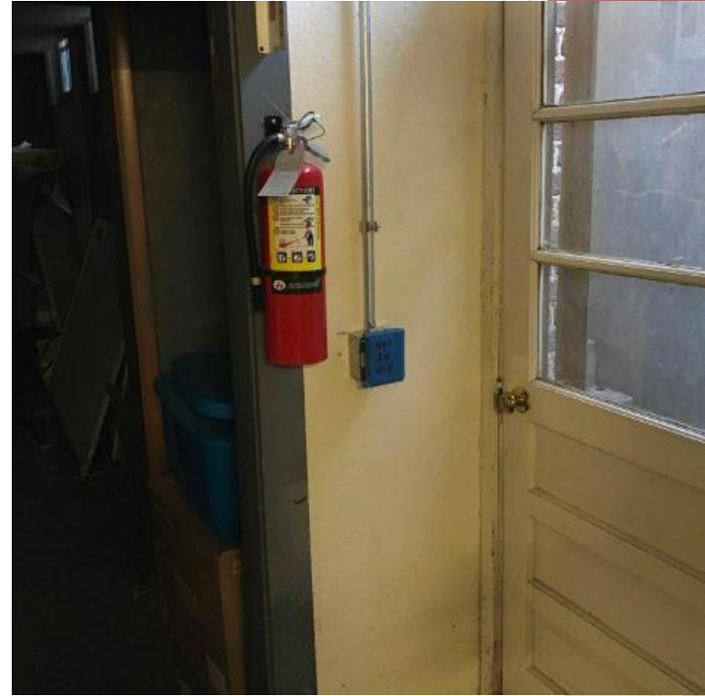
Installation of new fire alarm devices within existing building
