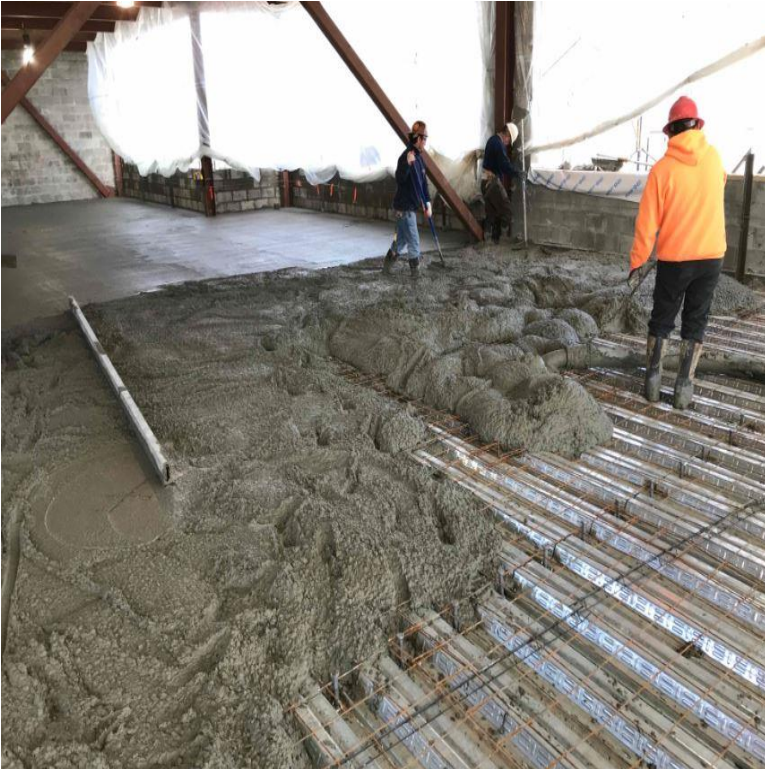
Second floor (Fifth Grade wing) concrete slab on deck
