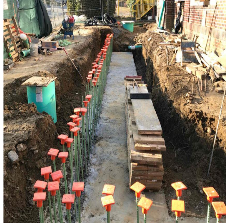
Poured footing for exterior ramp at Sage Terrace
