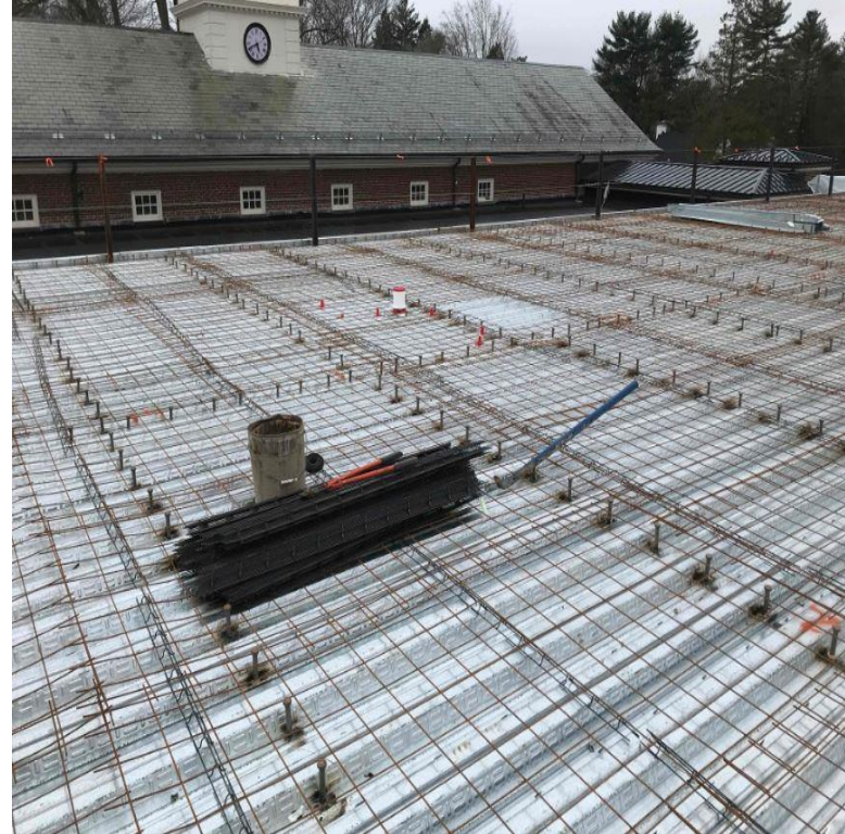
Preparation of roof deck above second floor Fifth Grade wing
