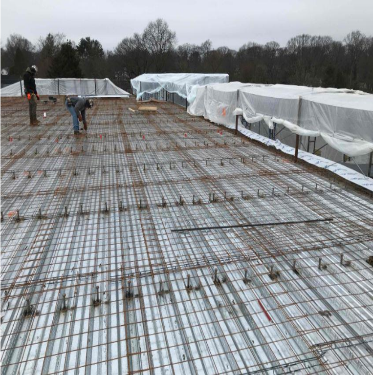
Preparation of roof deck above second floor Fifth Grade wing
