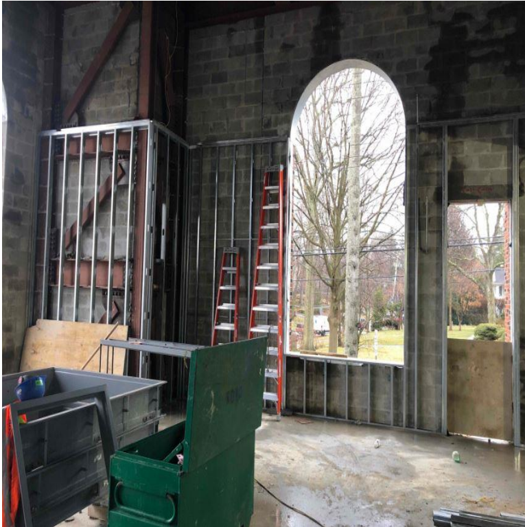
Construction of light gauge metal frame interior partitions at Learning Commons 146
