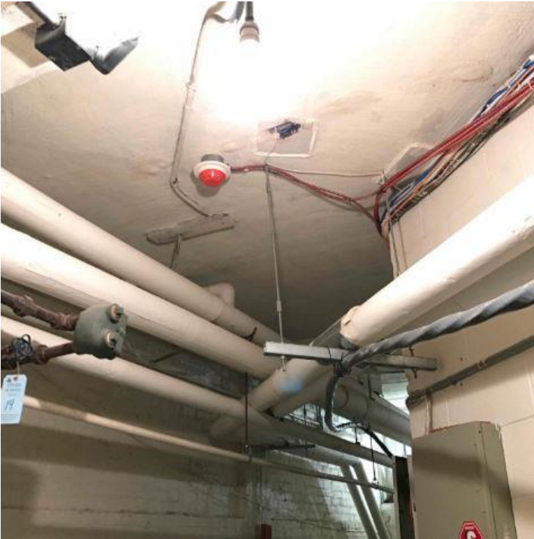
Installation of new fire alarm devices within existing building
