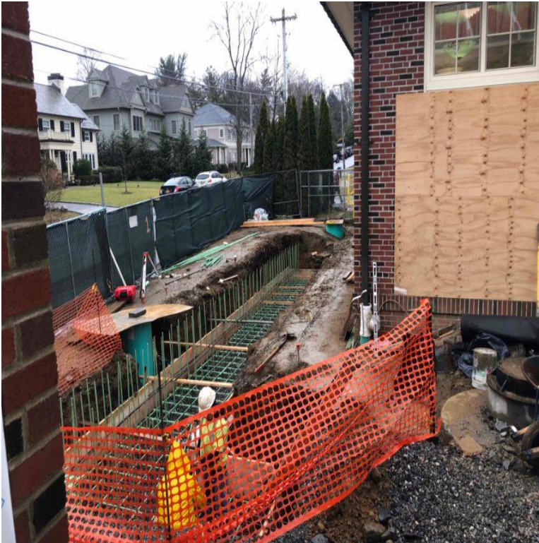
Installation of rebar for exterior ramp footing at Sage Terrace
