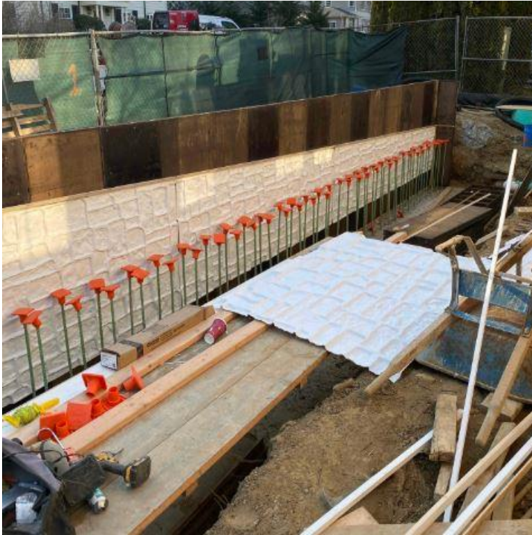
Installation of form lining for stamped concrete ramp walls at Sage Terrace
