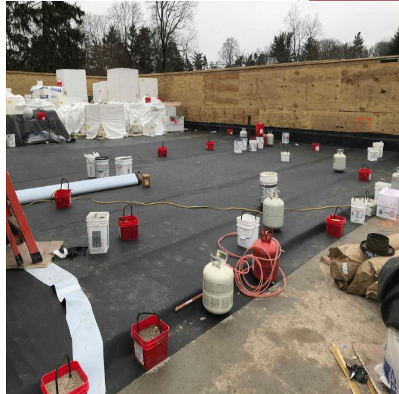
Installation of EPDM roofing system above Learning Commons and MPR areas.
