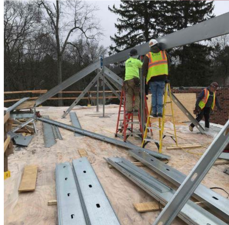
Construction of light gauge metal framing mansard roof above Learning Commons an MPR areas.
