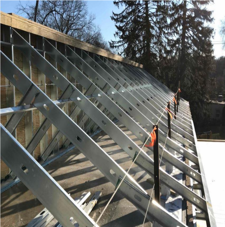
Construction of light gauge metal framing mansard roof above Learning Commons an MPR areas.
