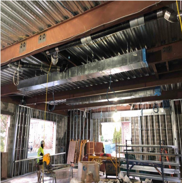
Installation of HVAC duct work at MPR Room 145
