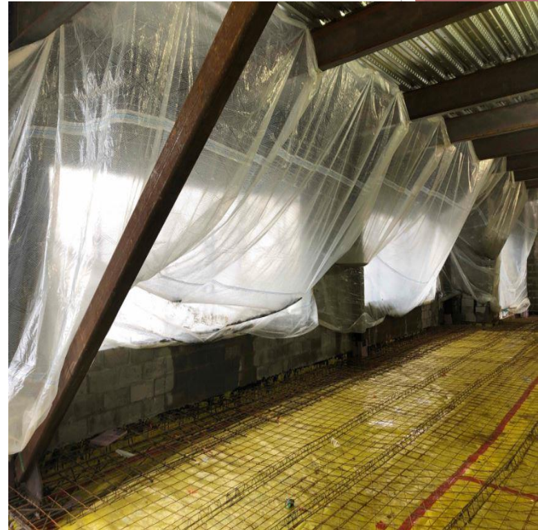
First floor slab on grade preparation
