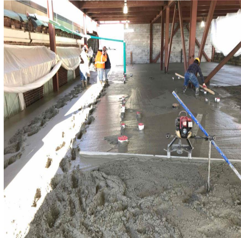
Second floor (Fifth Grade wing) concrete slab on deck
