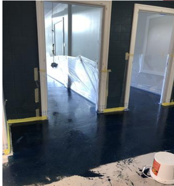
Preparation of slab for new flooring finishes at 2 nd floor of new addition
