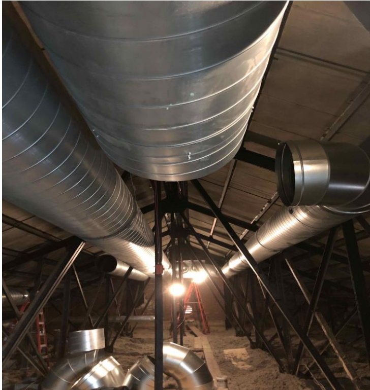
Installation of new duct work within existing attic (F.M.)
