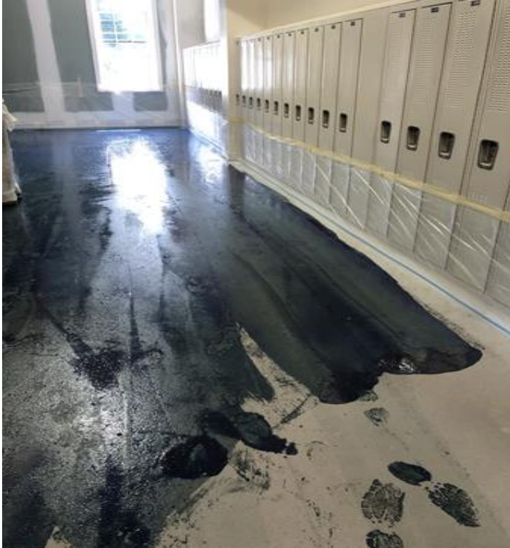
Preparation of slab for new flooring finishes at 2 nd floor of new addition
