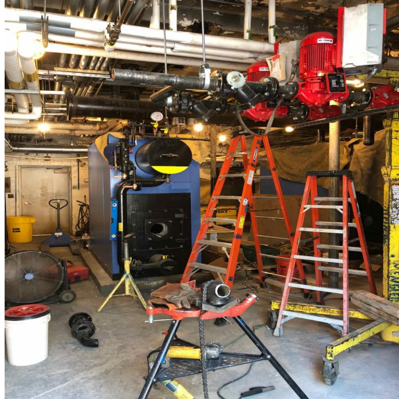
Installation of new boilers (E.W.)
