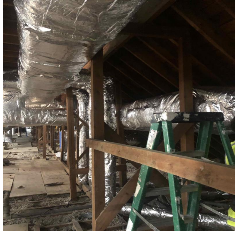
Installation of new duct work within existing attic (E.W.)
