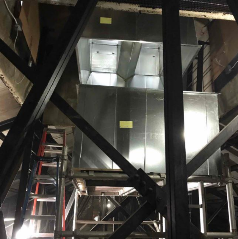
Installation of new duct work within existing attic (F.M.)
