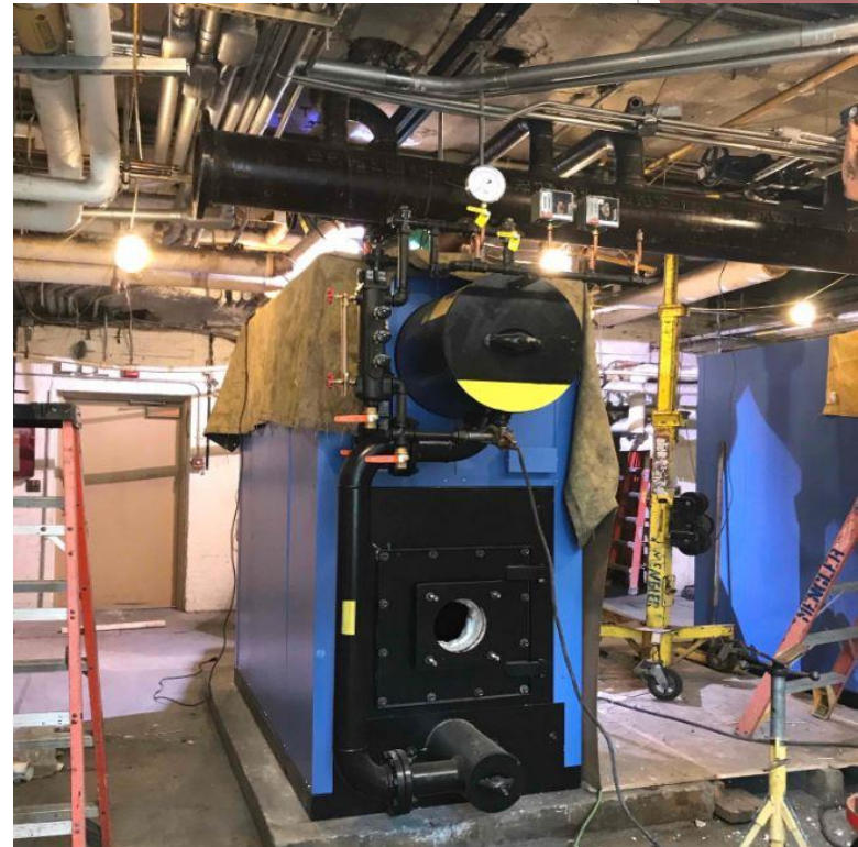
Installation of new boilers (E.W.)
