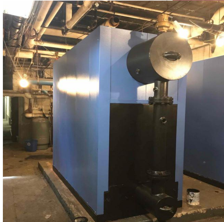
Installation of new boilers (F.M.)
