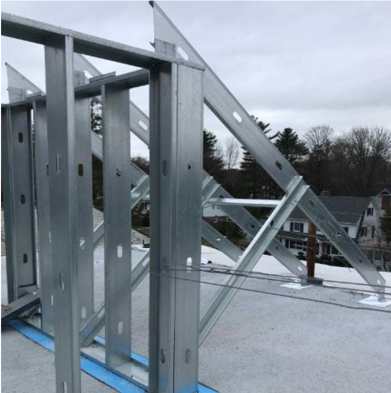
Construction light gauge metal mansard roof framing
