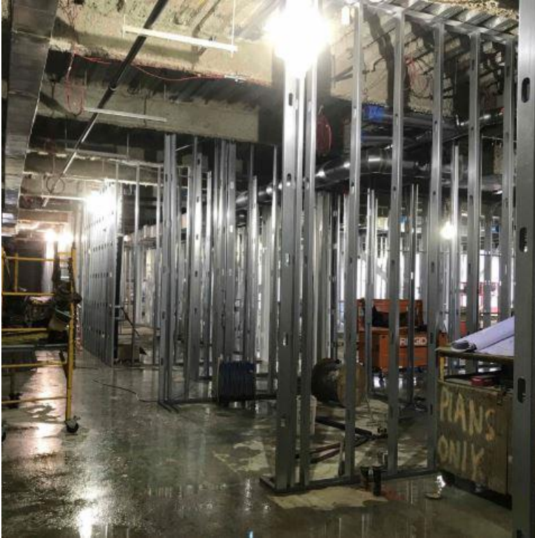
Proposed interior light gauge metal partition framing
