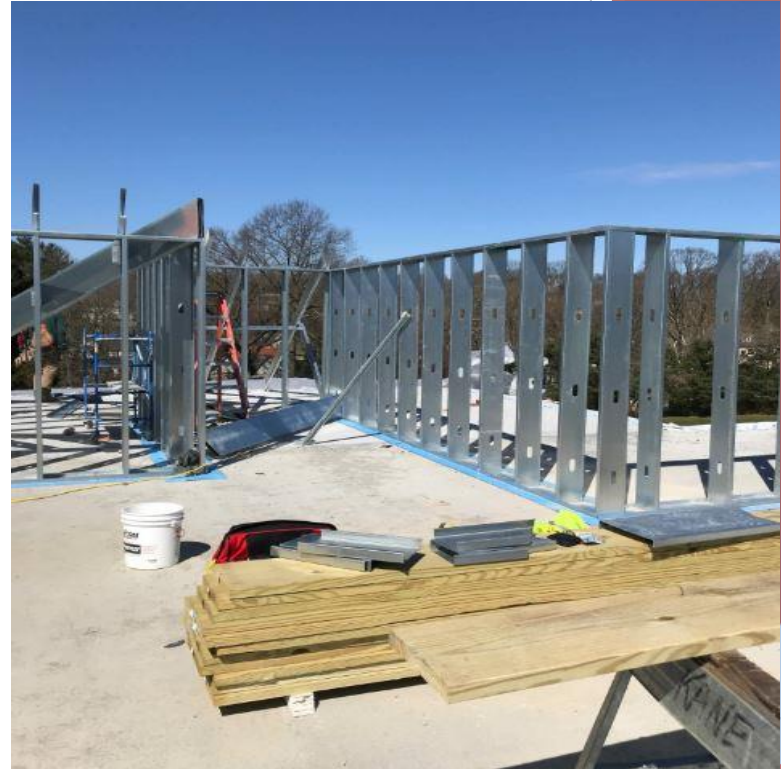
Construction light gauge metal mansard roof framing
