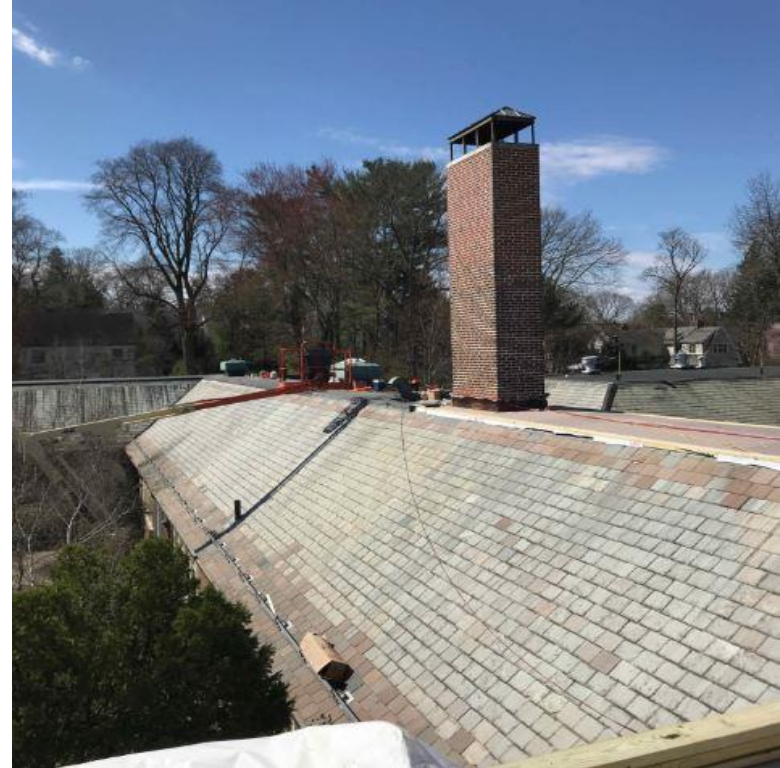
Replacement of existing roofing system adjacent to Sage Terrace
