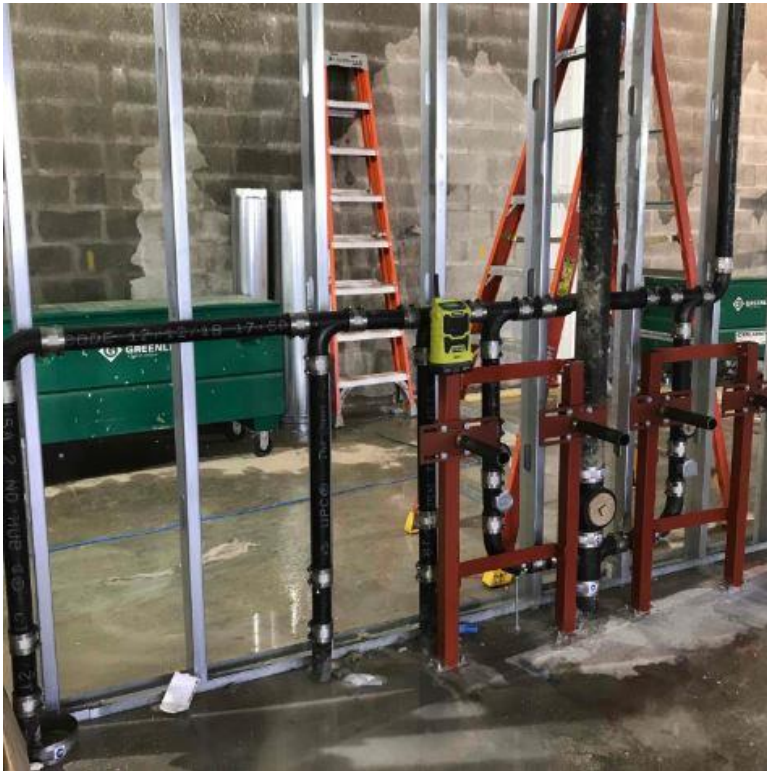
Proposed bathroom plumbing roughing
