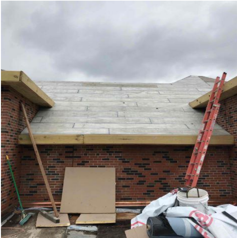
Installation of concrete roof planking
