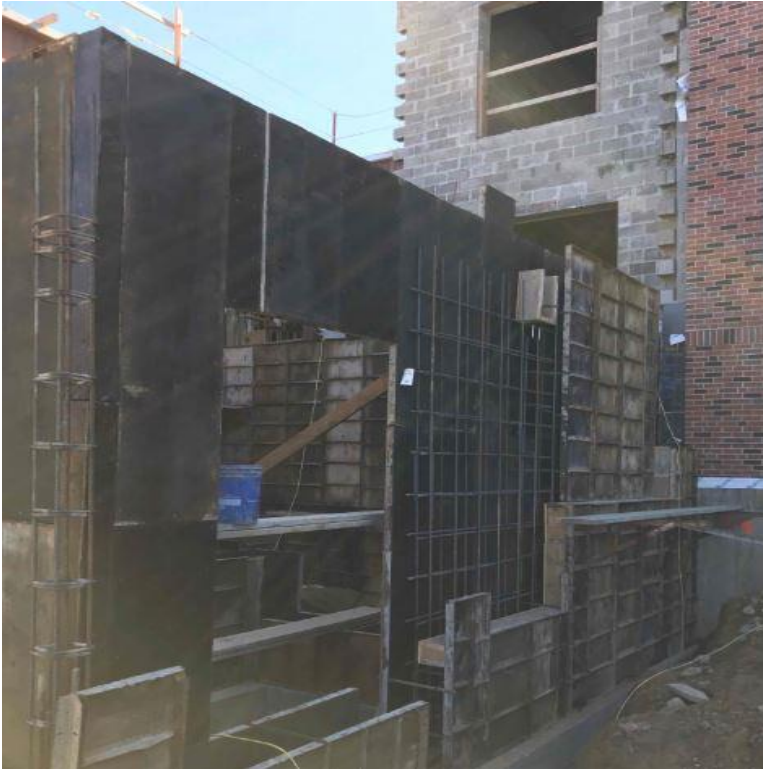
Construction of foundation formwork and rebar at proposed stair well 153
