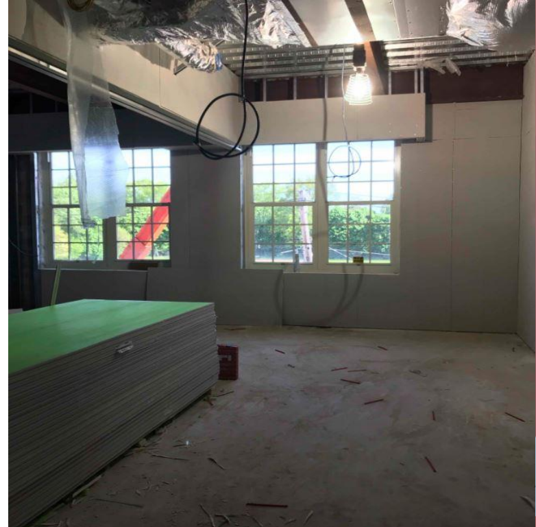
Installation of Sheetrock Wall Finishes at 1 st Floor of New Addition
