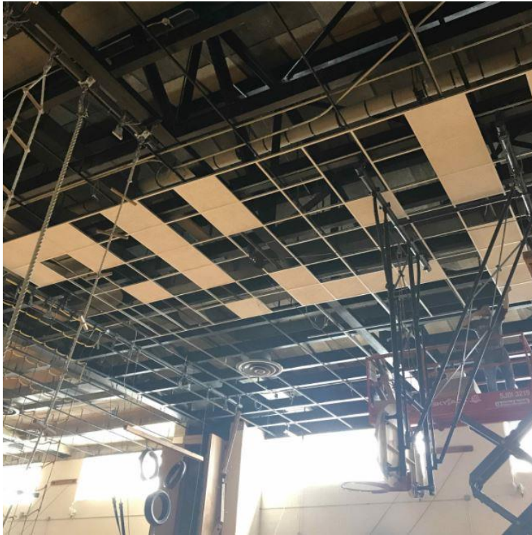
Installation of new ceiling grid and tiles within Middle School gymnasium.
