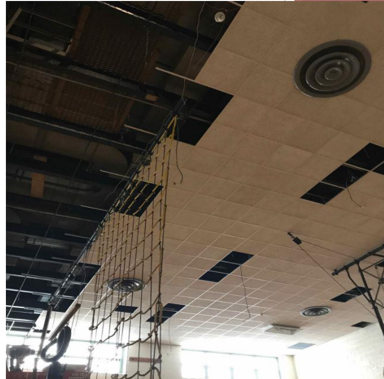
Installation of new ceiling grid and tiles within Middle School gymnasium.
