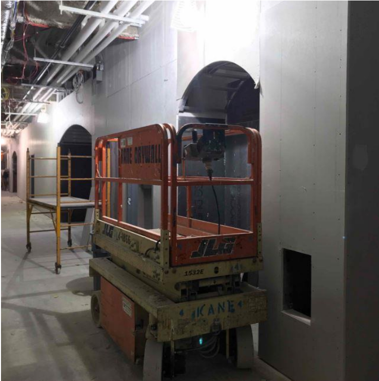
Installation of Sheetrock Wall Finishes at 1 st Floor of New Addition
