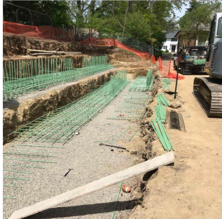
Construction of concrete ramp/retaining wall.
