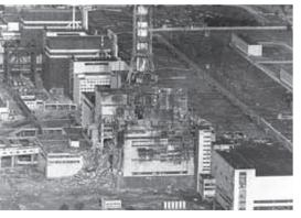
During a test at the Chernobyl nuclear power plant, the emergency protection system was turned off. The reactor overheated, causing an explosion.
